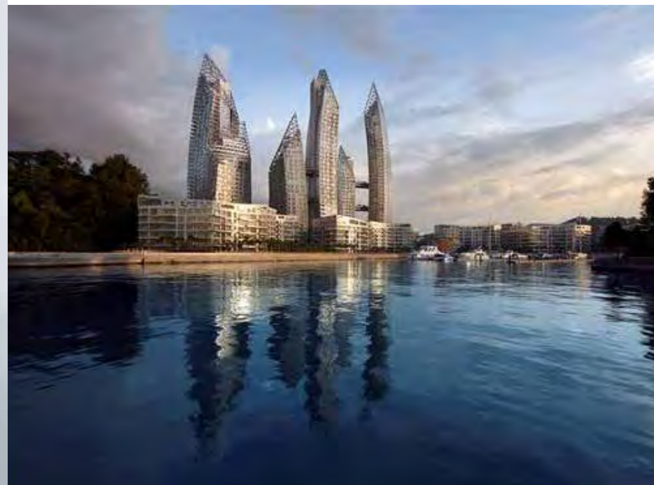
Reflections at Keppel Bay
