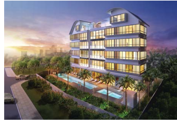
833 MB Residences (Construction in progress)
