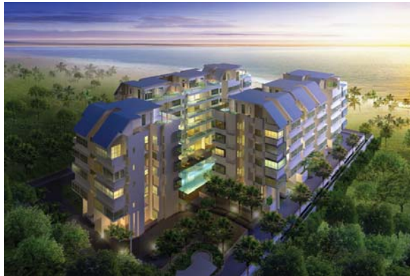
Coastal Breeze Residences (Construction in progress)
