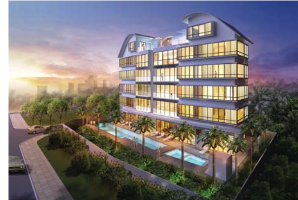
833 MB Residences (Construction in progress)
