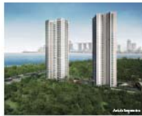
The Meyerzie (under construction) • Meyer Road • 299 units Expected Date of Vacant Possession No later than 1 Oct 2016
